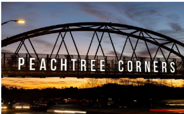
Pedestrian bridge example
