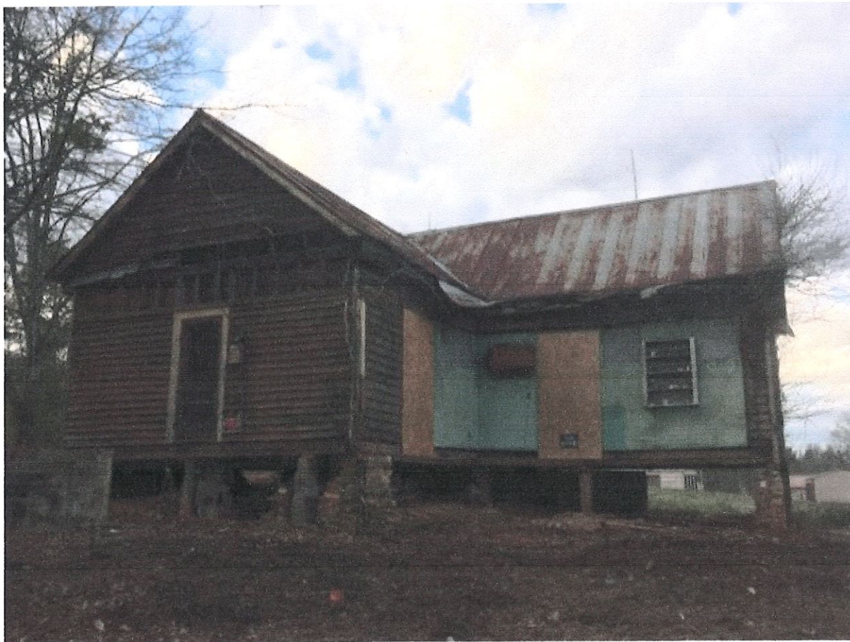
Above photo of the house from the Southeast corner
