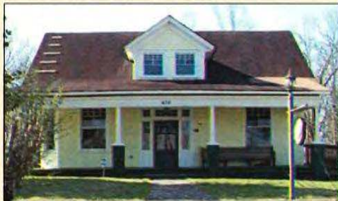
The gabled dormer within the roofline of this Arts and Crafts Style home is true to the original design.
