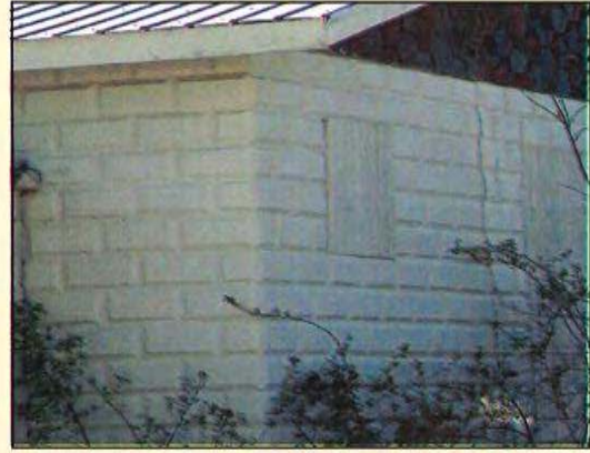
Cast concrete blocks have been in use since the early 20 th century
