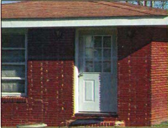
Flagcrete masonry is a unique building material used during the 1950s and 1960s
