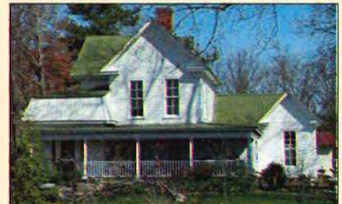
Almost completely intact, the roofline of this Folk Victorian home has been modified with a mansard addition that is more commonly associated with the Second Empire or Beaux Arts Styles.
